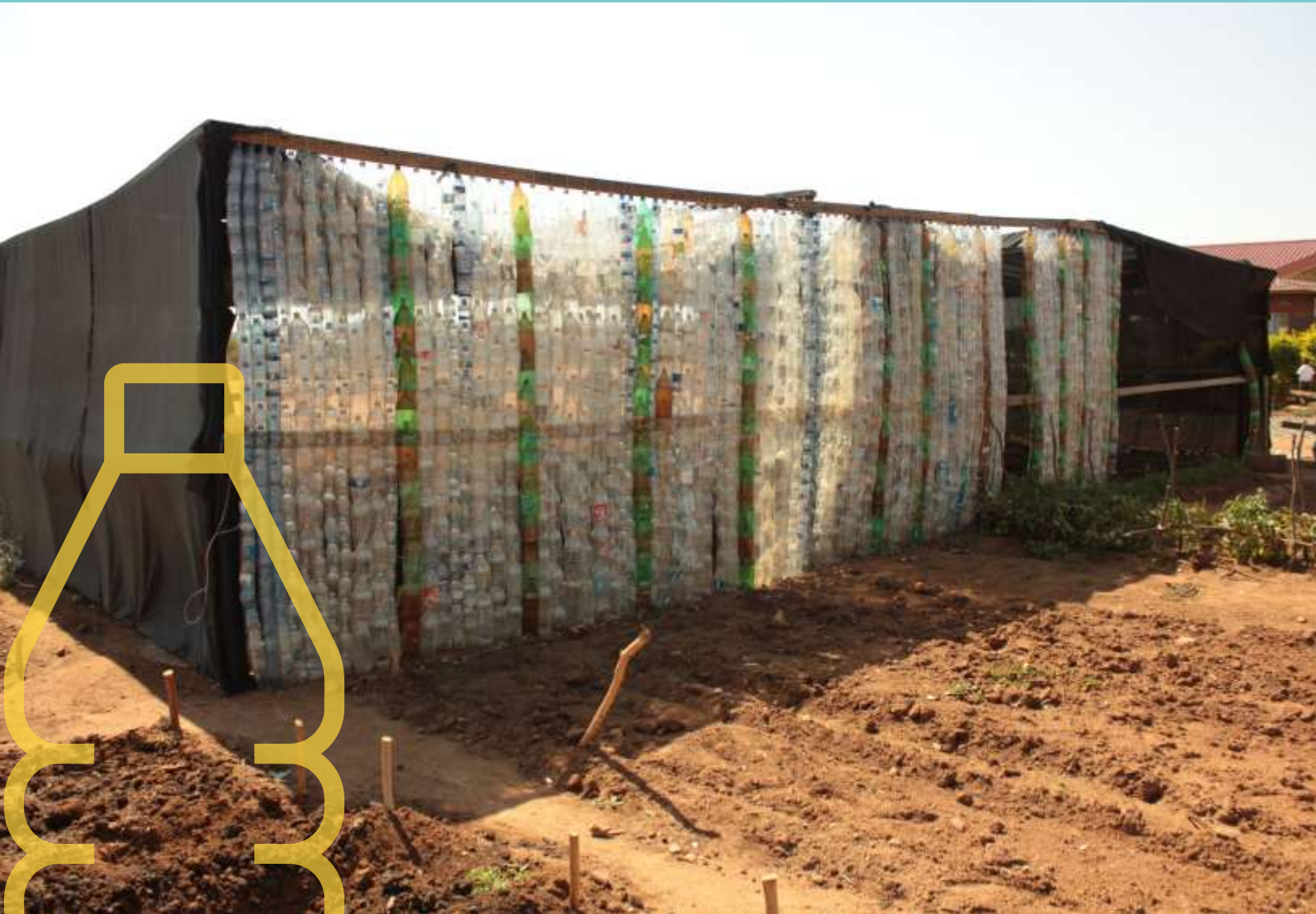
Plastic bottles collected during a clean-up action turning into a greenhouse wall
